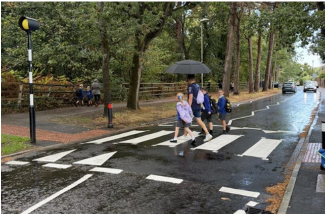
New pedestrian crossing on Sandy Lane
